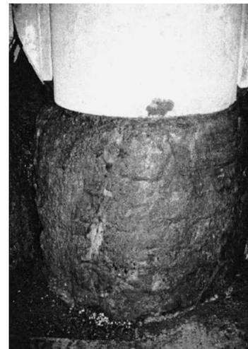
Photo 5 Joint between steel pipe (upper part) and cast-in-place concrete pile (lower part)
