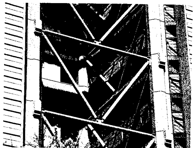
Photo 2 Appearance of pin joint type bracing
