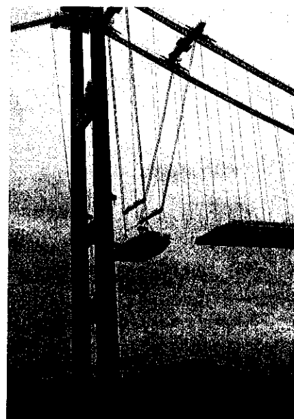
Photo 4 Stiffening girder under the swing erection
