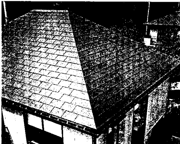
Photo 2 Work example of "River Shingle"
