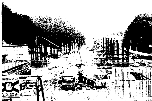
Photo 3 Applying SEED-Form to pier in Kashiwagidani Bridge
