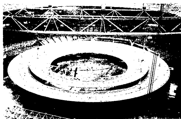
Photo 2 Application of KT-Truss and tension member
