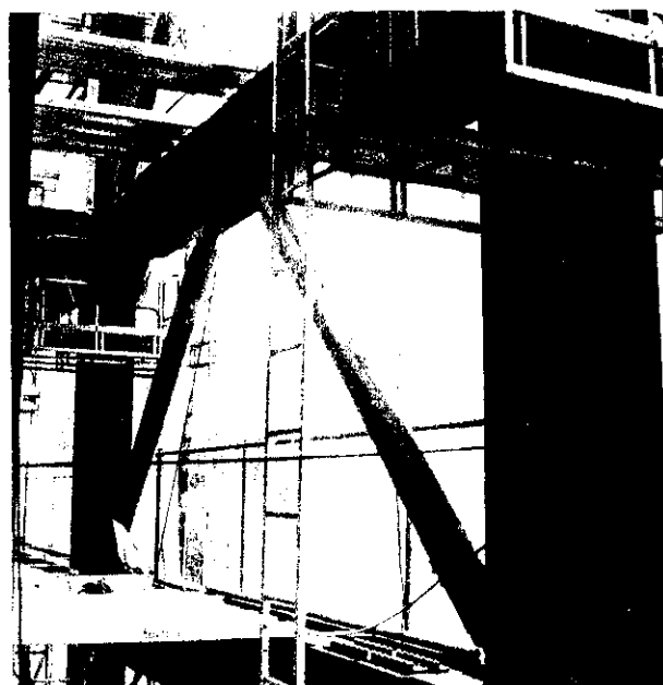
Photo 3 Application of FLD member
