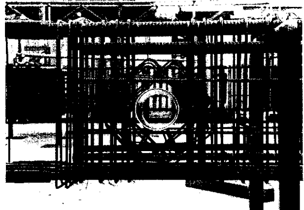
Photo 5 Riverren during bar arrangement
