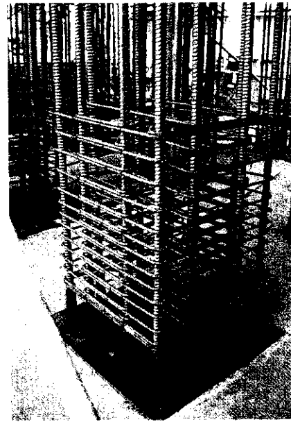
Photo 4 Riverbon Multi Spiral Hoop during bar arrangement
