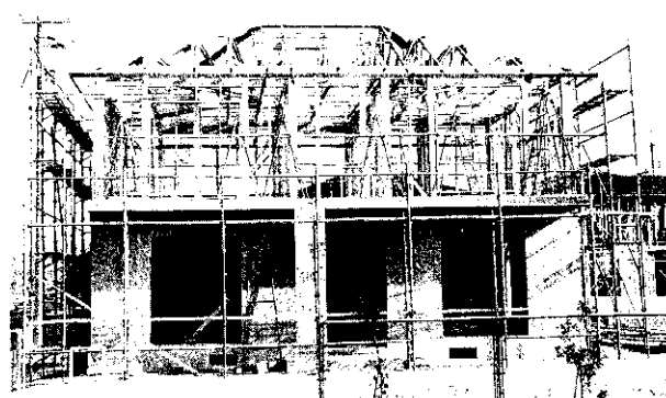
Photo 1 Light gauge steel framing of residence
