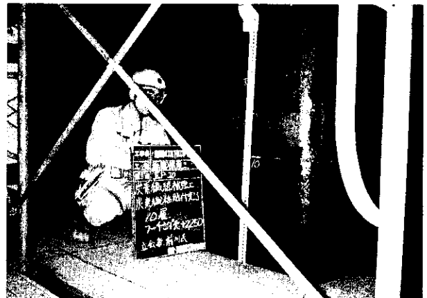
Photo 5 Reinforced pier by carbon fiber
