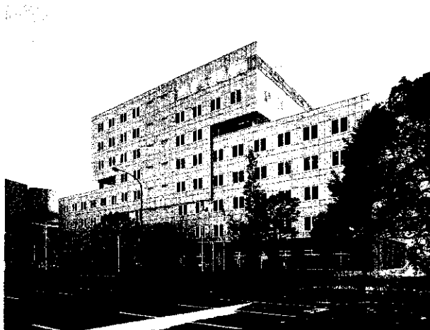
Photo 3 Outside view of new Kobe Head Office
