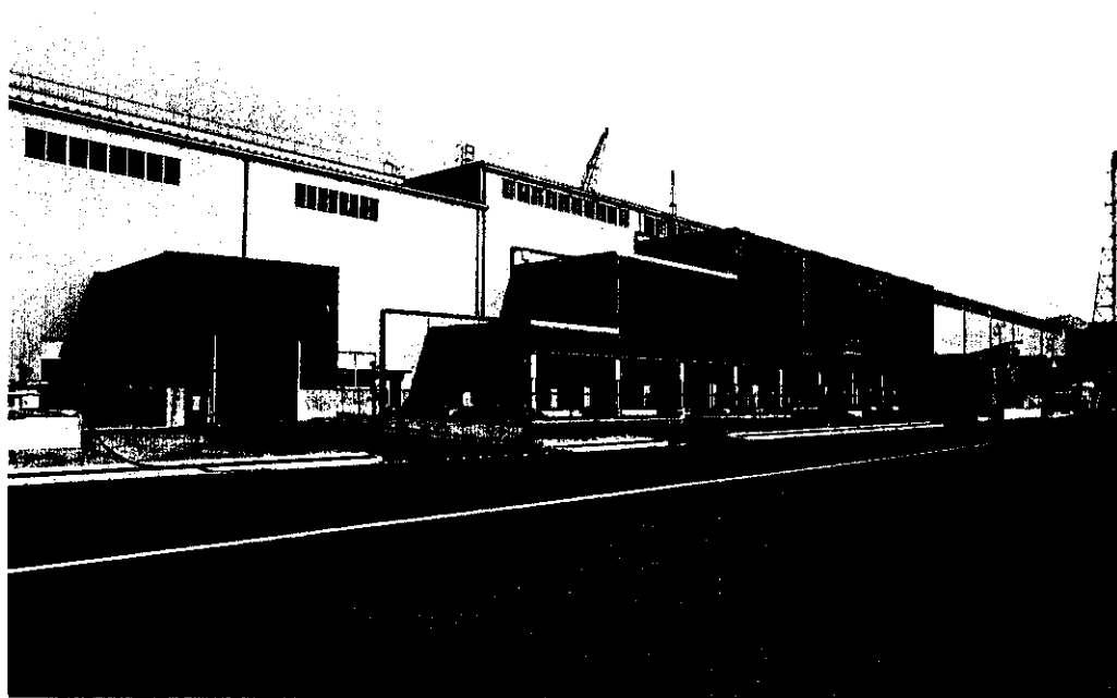
Photo 3 Hot finishing plant from west side
