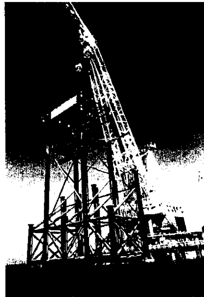
Photo 1 Installation of the jacket for the Kisarazu Man-Made Island
