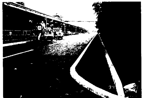
Photo 4 Road paved by asphalt concrete containing slag
