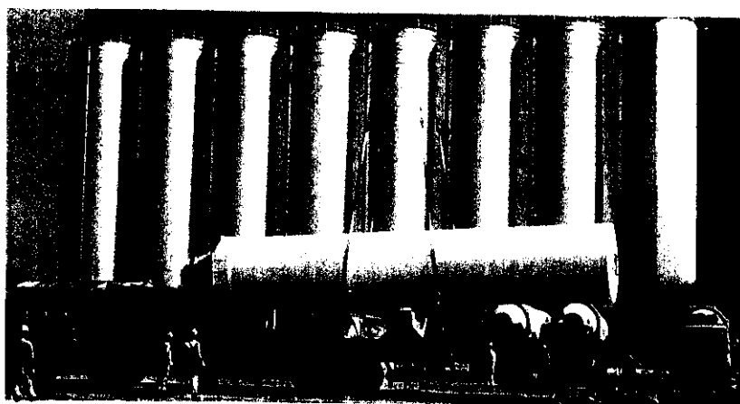
Photo 5 12-m length silo in construction field (made of the pipe shown in photo 4)
