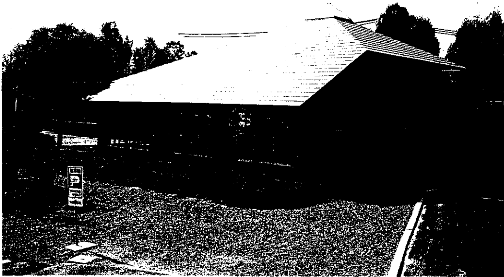
Photo 2 Example of RESINO 15-GF applied roofing
