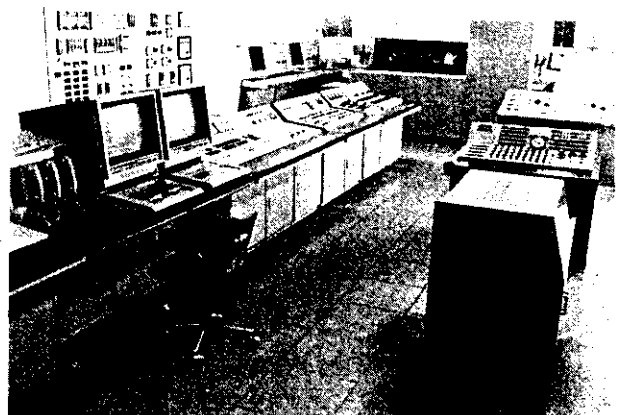
Photo 1 Central control room
