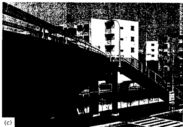
(a) Roof (b) Bridge (c) Footpath bridge
