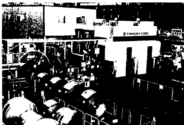
Photo 1 View of entry section
