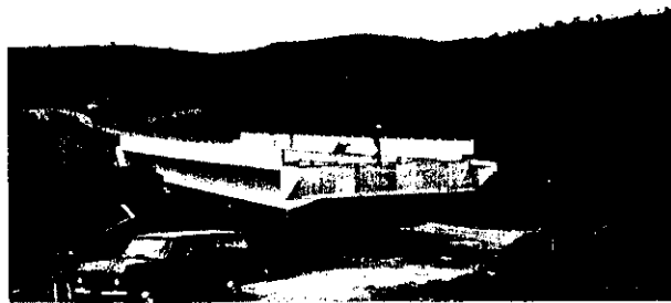
Photo. 3 Concrete bridge of Rio Maracuja (Under construction June, 1980)
