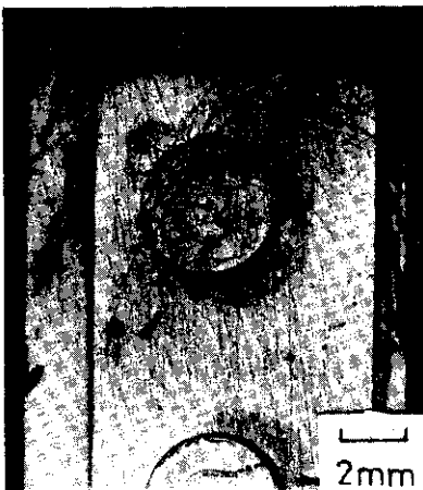
Photo. 4 Typical appearance of stress corrosion cracking in spot welded specimen of Type 304 stainless steel after 11 weeks test in 21 000ppm Cl - solution at 80°C
