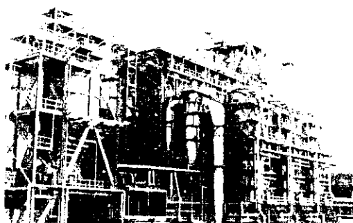
Photo. 1 General view of CDQ plant
