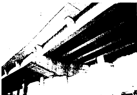
Photo. 2 Completed HPC composite girder
