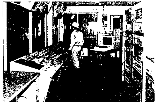
Photo. 4 Interior of the operating room
