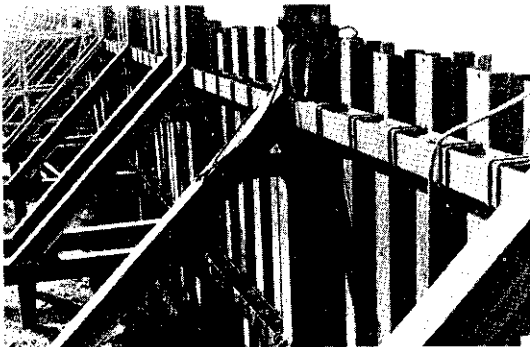
Photo. 9 Driven sheet piles fixed to steel blocks by U bolts (K·H B type)
