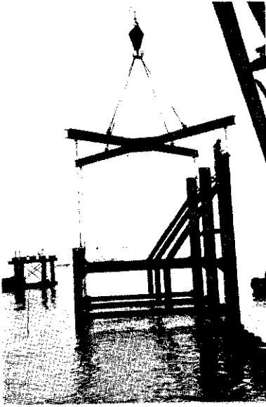
Photo. 4 Hanger of steel block at work
