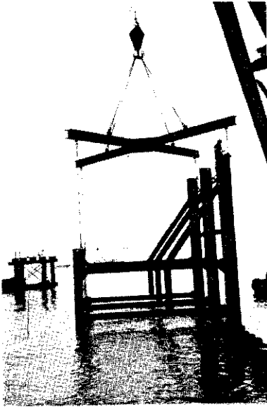
Photo. 4 Hanger of steel block at work
