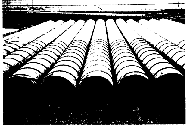
Photo 26 Rotary penetration steel pipe pile (drill pile method)
