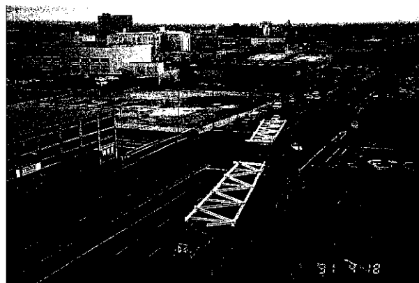
Photo 2 Transportation of truss
