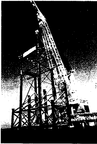
Photo 1 Installation of the jacket for the Kisarazu Man-Made Island
