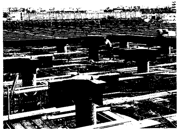
Photo 5 Installation of pile heads by ordinary method
