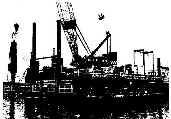
Photo 4 STEP method over the flood-regulating reservoir
