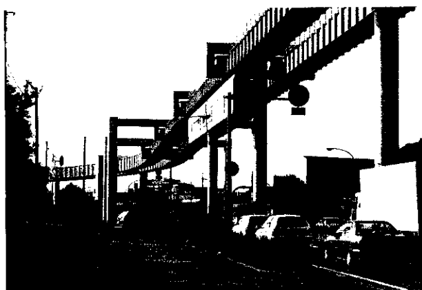
Photo 5 Suspension type monorail structure
