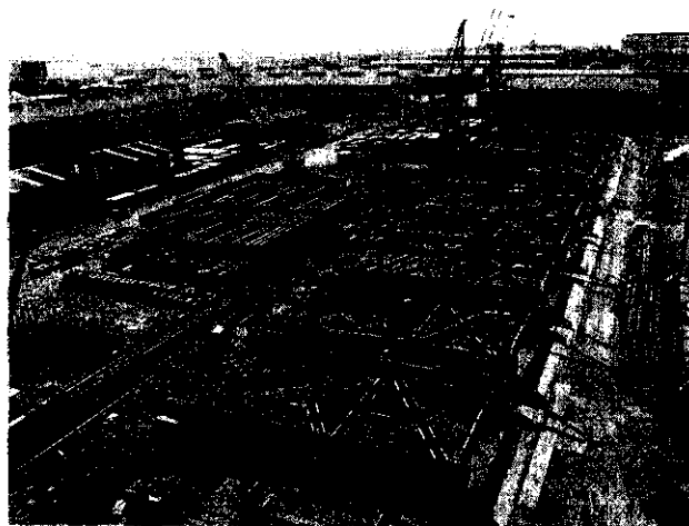
Photo 1 Panel assembly of jacket at Harima fabrication yard
