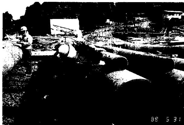
Photo 1 Site fabrication of interlocked steel pipe piles
