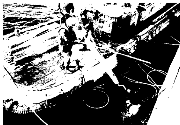
Photo 2 Aluminum alloy anode installation
