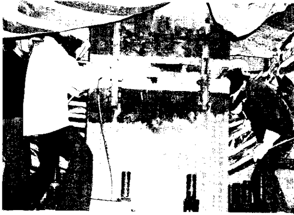
Photo 5 Field welding of column-to-column connection
