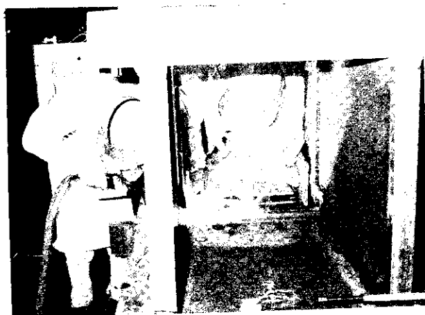
Photo 4 Welding lower flange of girder
