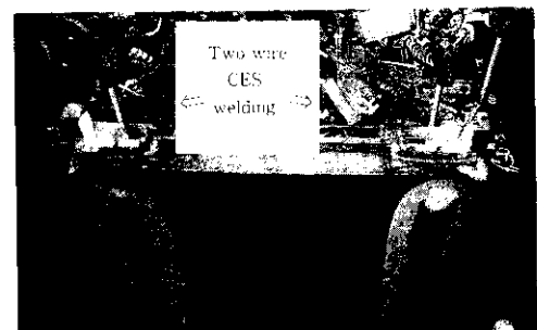
Photo 2 Two wire CES welding for column-to-girder joints
