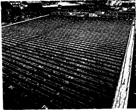
Photo 1 Steel girder erection for the top slab of the Mukaihara Tunnel
