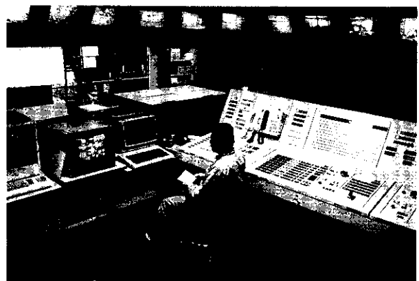
Photo 1 View of yard control pulpit
