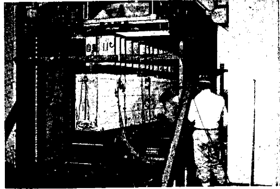
Photo. 3 Setup for flexure test on SC beam with deformed flange H-shapes
